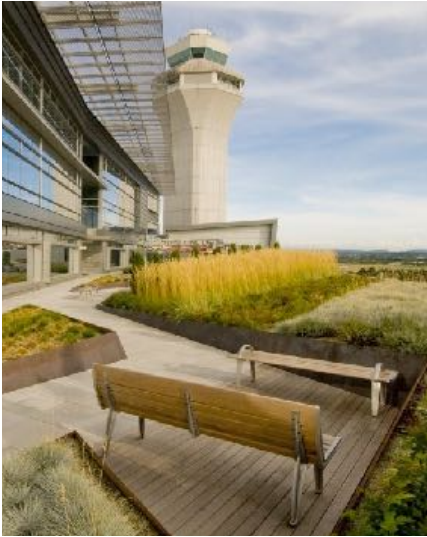
port of portland headquarters Living Machine® System
